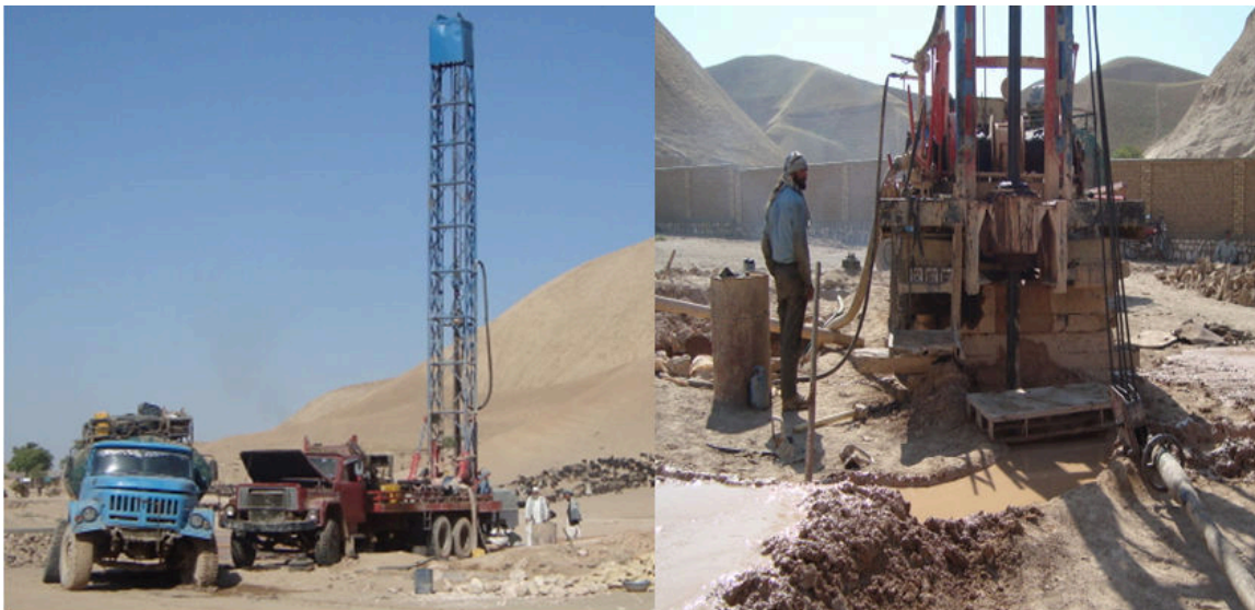
Fig. 26 Gul Quduq village exploration well drilling process
