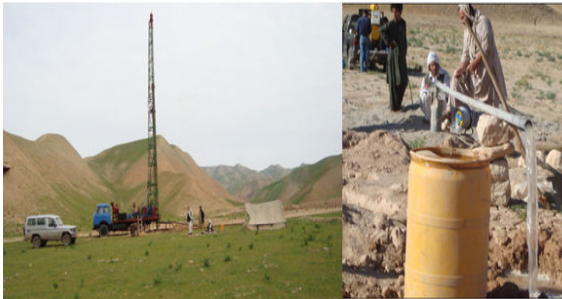
Fig. 24, Drilling process of exploration well in Mahad village
