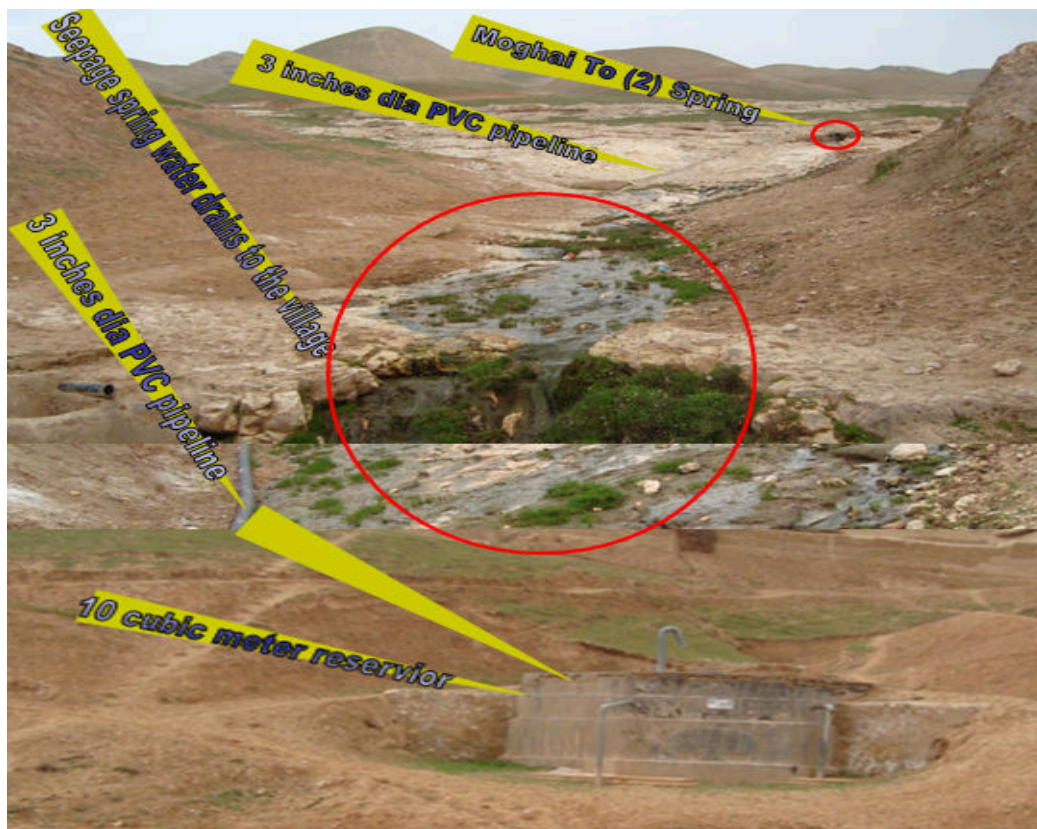
Fig.29. Moghai To (2) spring and reservoir location
