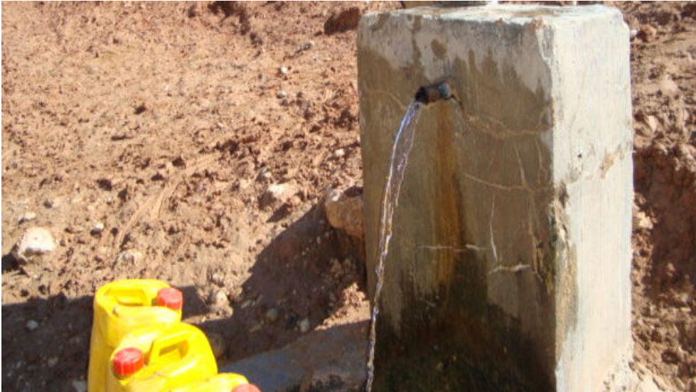
Fig.30 Feature of water wastage from a stand post without tap
